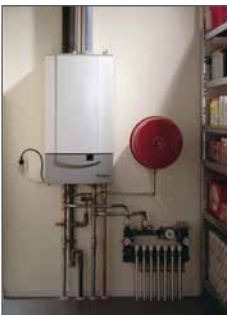
(Afb. 1) Cv-ketel opstelling.
